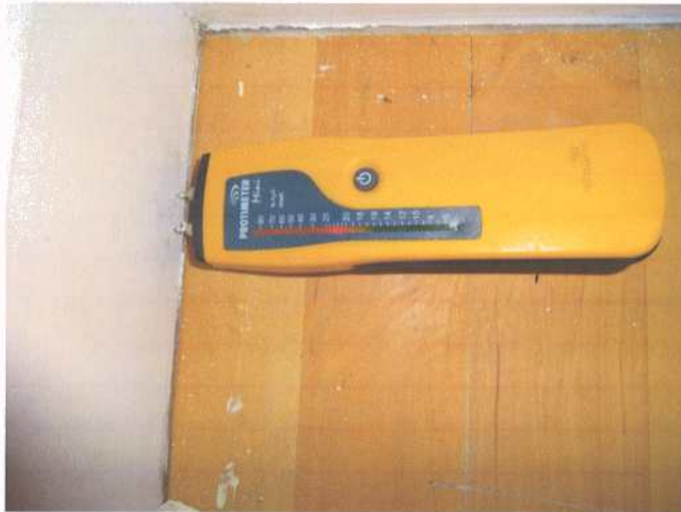
Bedroom 1 reading 24% moisture recorded
