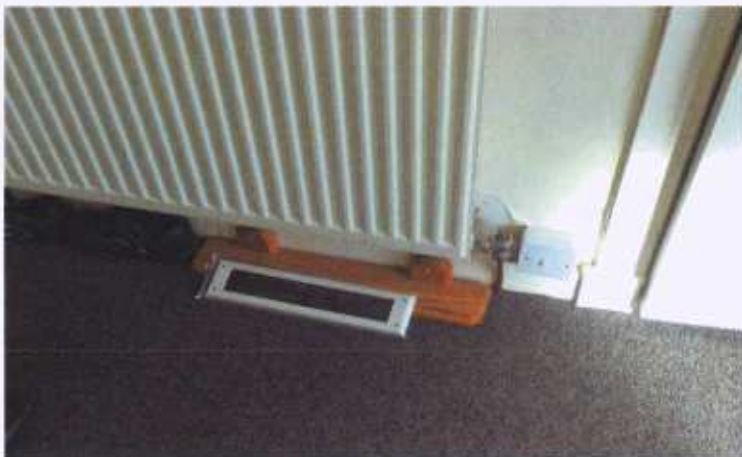
Photograph 3 :- Missing TRV 2
