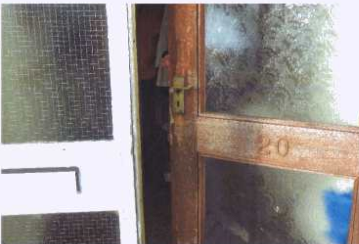
Photograph 6 :- Front entry door and surround
