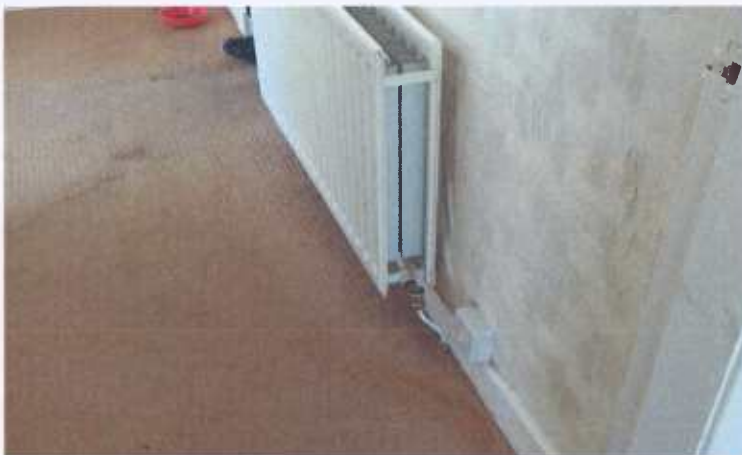
Photograph 2 :- Missing TRV 1
