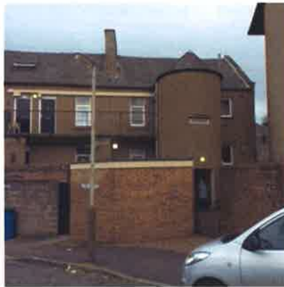
Mid Road elevation – 13 September 2016
