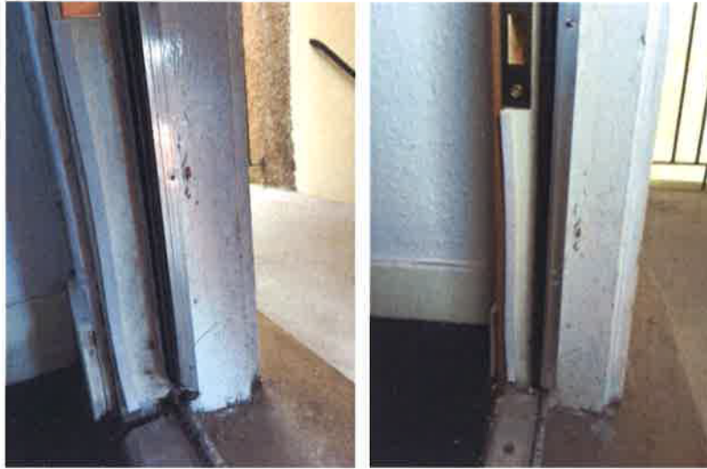
Front door frame – 20 June 2016 Front door frame – 13 September 2016
