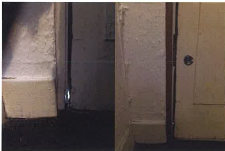
Front door frame (inside) 20 June 2016
