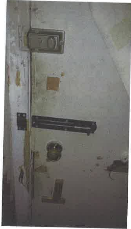
Photo 2 – Functioning door locks
