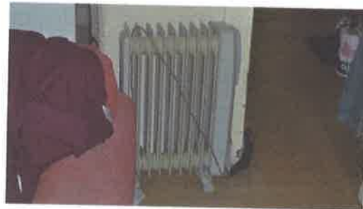
Photo 7 – Expired electric heater
