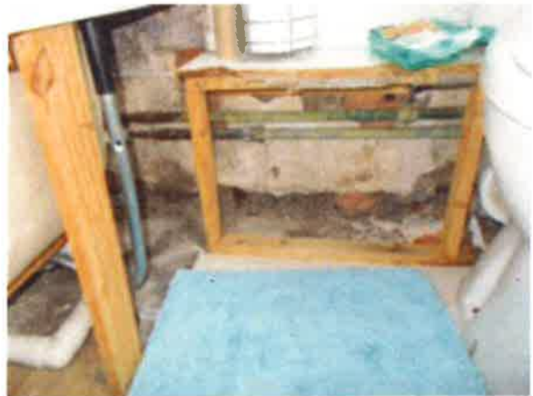
Bathroom - pipes exposed following emergency repair - boxing removed
