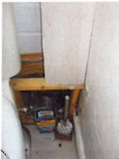
Bathroom - pipes exposed following emergency repair - boxing removed
