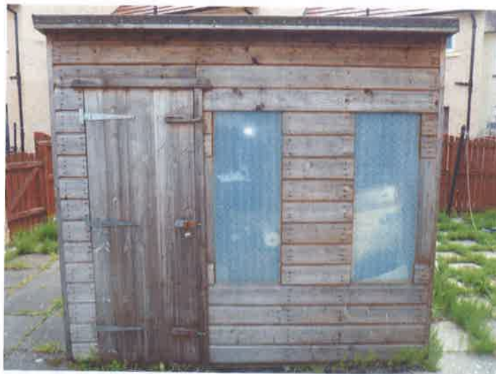
20. Landlord's shed in Garden
