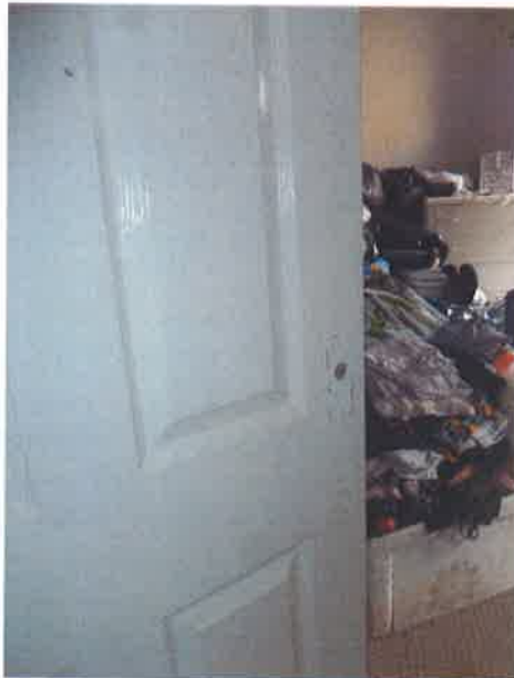
14. Missing handle at front bedroom door
