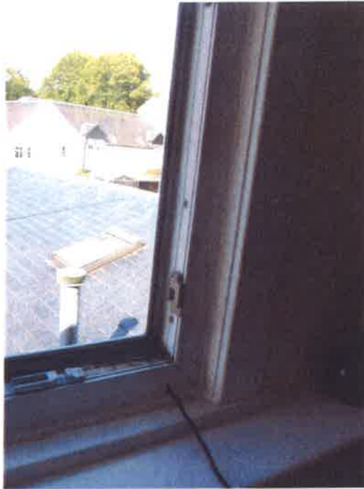
21, Repairs to window and cill in bathroom
