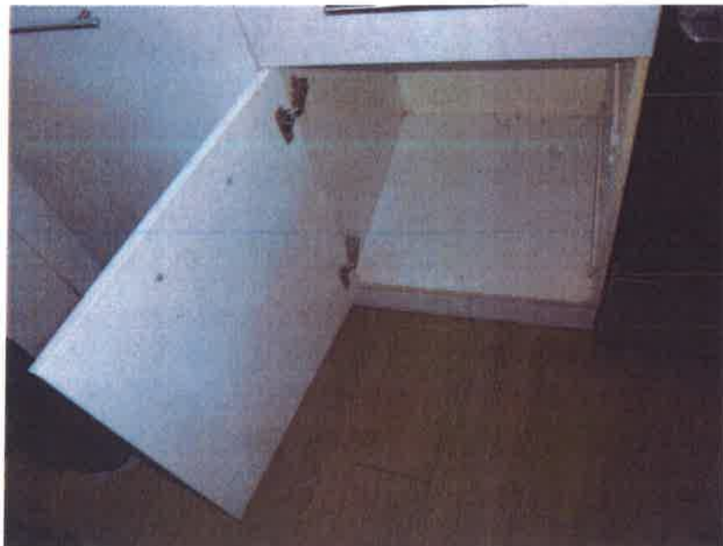
10. Repair to kitchen base unit hinges
