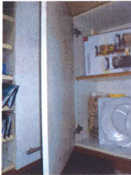
11. Repair to kitchen wall unit hinges
