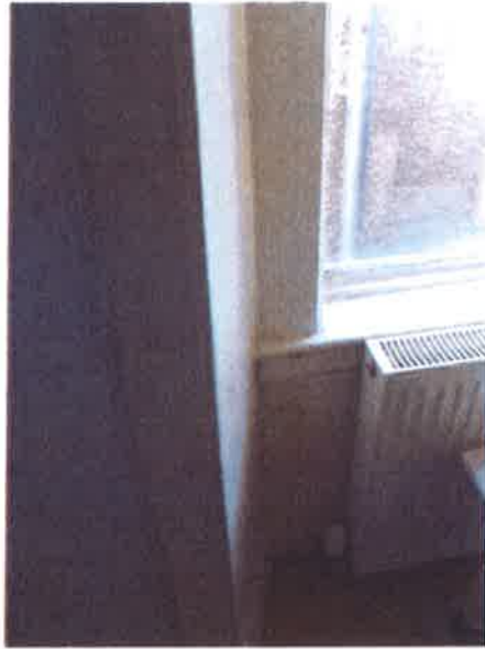
3. Living room window repair
