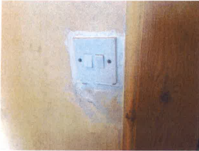
17. Replacement light switch in lower hall
