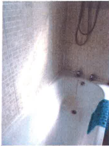
7. Tiled area and pointing at bath
