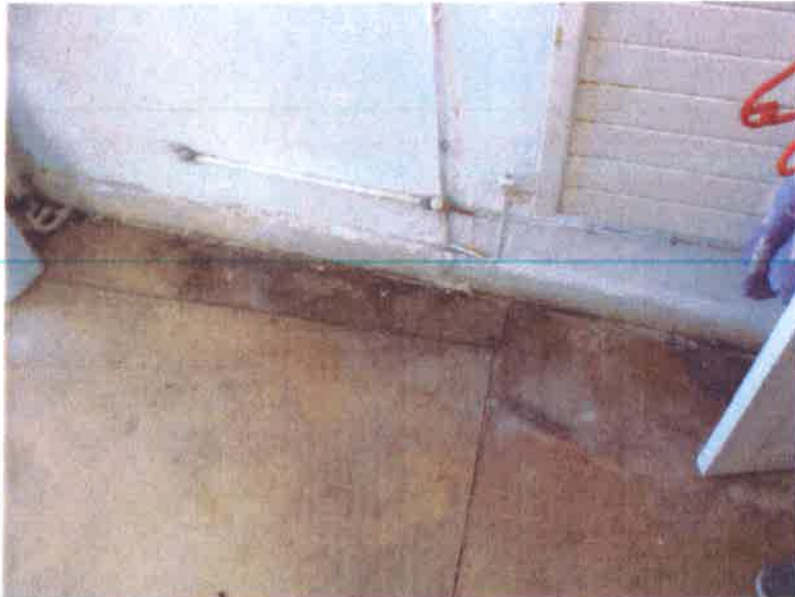
6. Central heating pipe repair in bathroom
