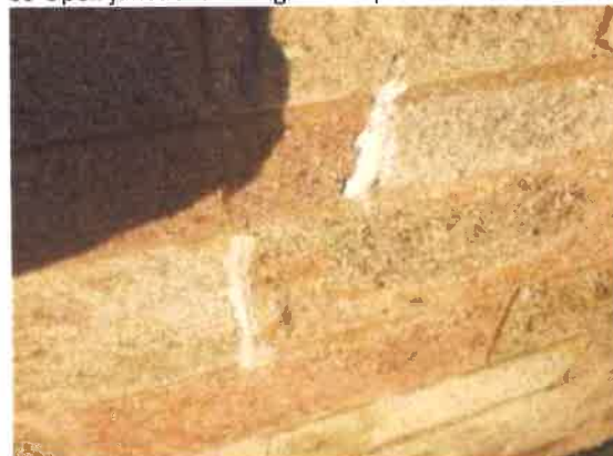
41 Patch pointing works.
