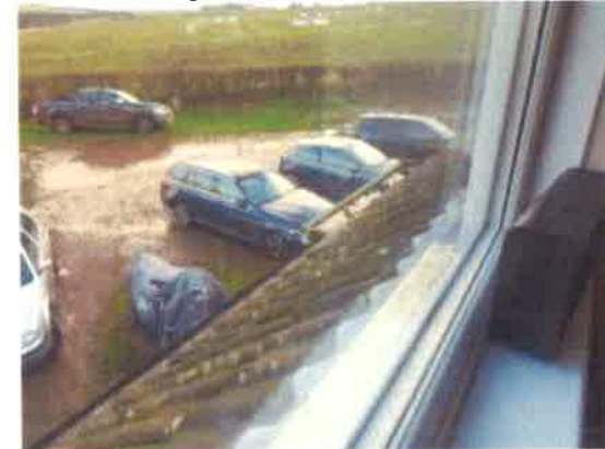
24 Roof covering viewed from dormer.
