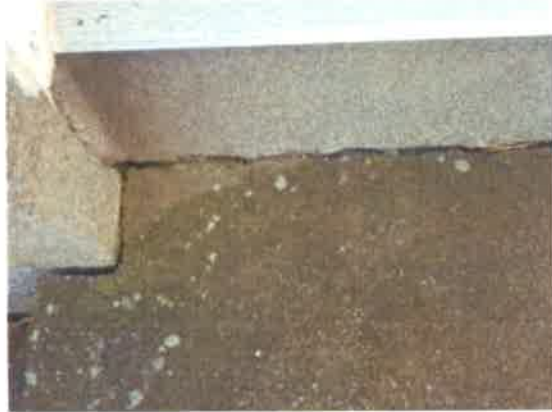
38 Open junctions with gable steps.
