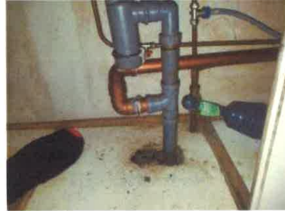
10 Pipework below sink.
