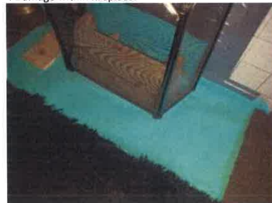
6 Temporary protection at hearth.
