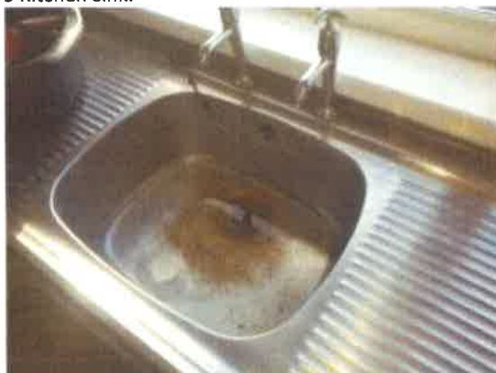
11 Blocked drainage at sink.
