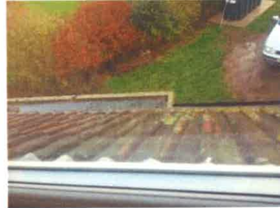
22 Roof covering viewed from dormer.
