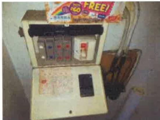
14 Consumer unit with rewirable fuses.
