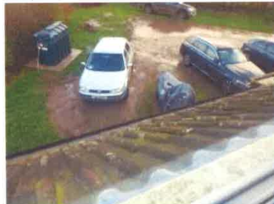
23 Roof covering viewed from dormer.
