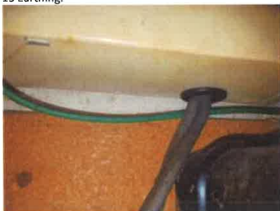
17 Cable entry and grommet.
