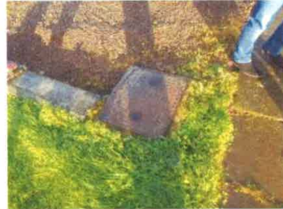
58 Inspection chamber.
