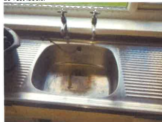
18 Drainage blockage.
