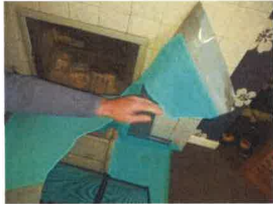
2 Temporary protection at fireplace.
