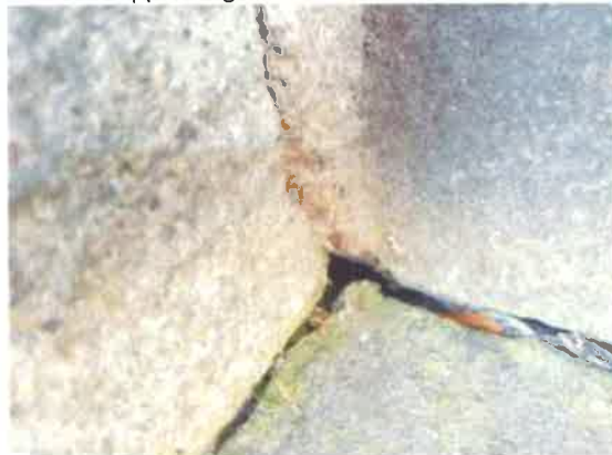
39 Open junctions with gable steps.
