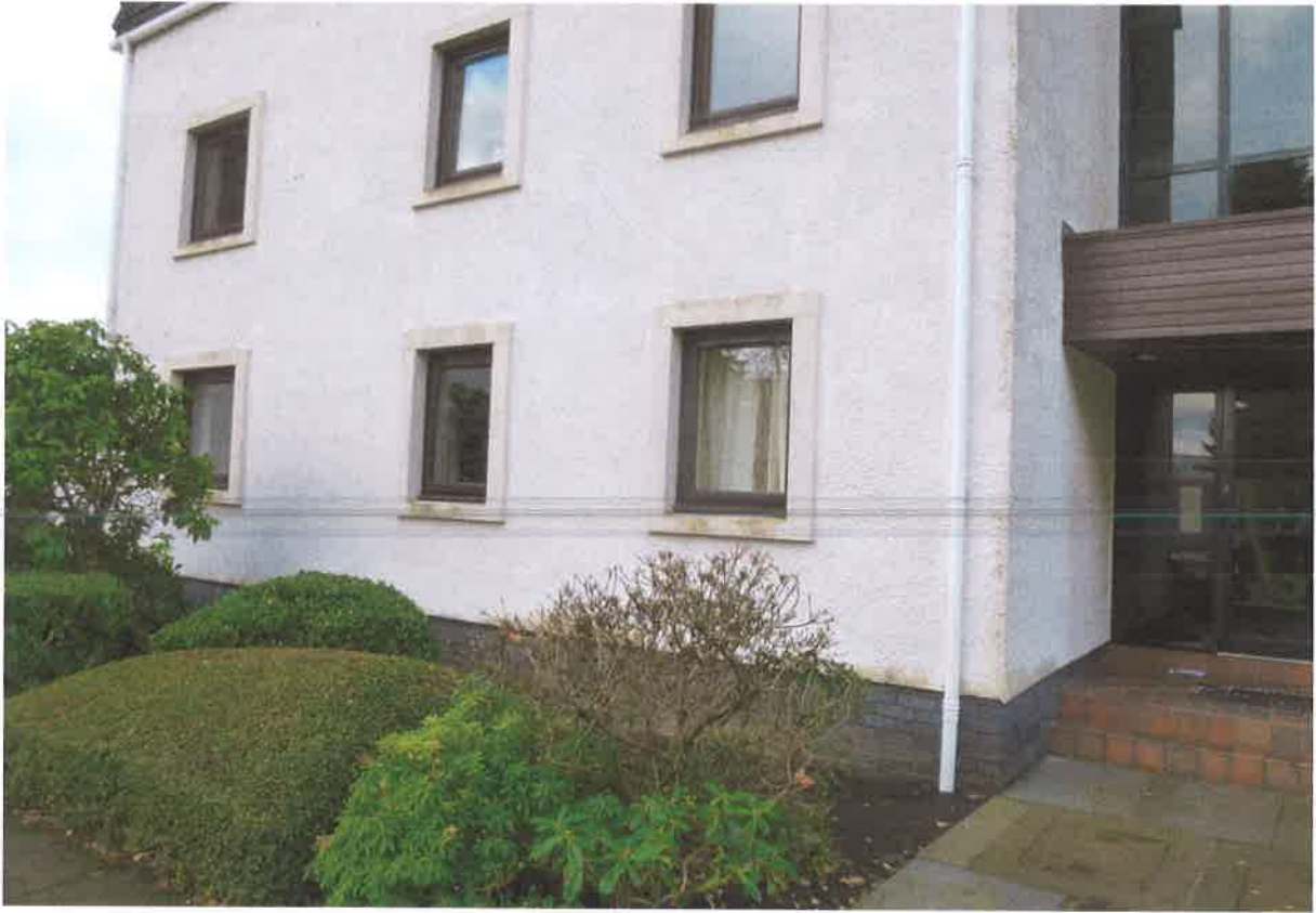
16 Guthrie Court – Front Elevation, Ground floor flat
