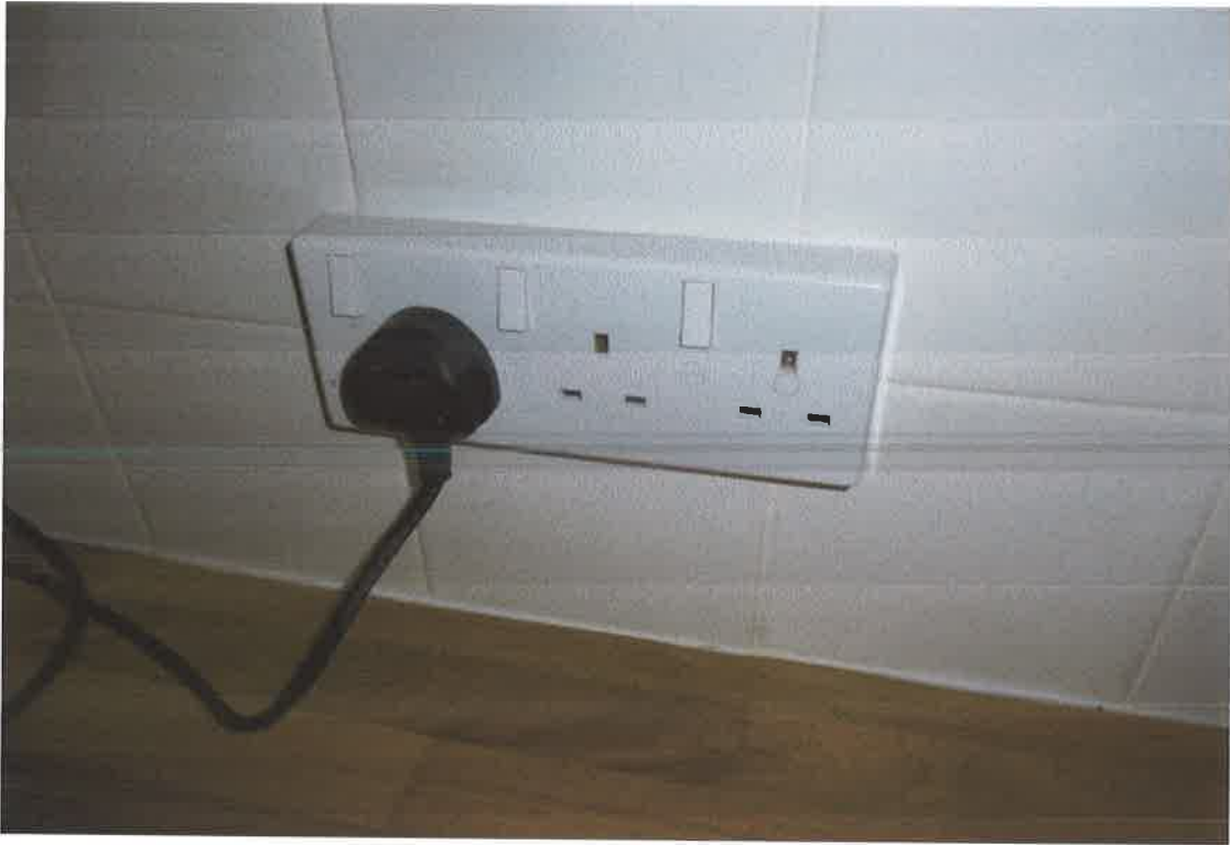
Kitchen – new electrical sockets
