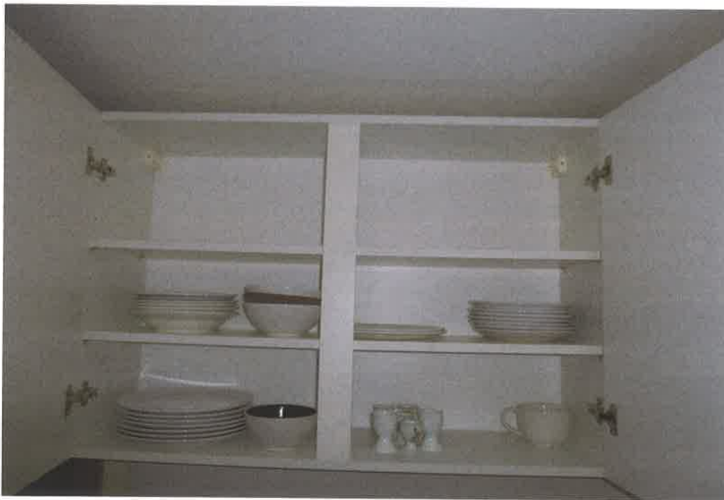
Kitchen units – no mould inside. Dry.
