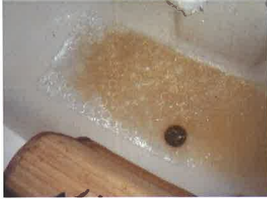
DISCOLOURED WATER AT SINK AND IN BATH
