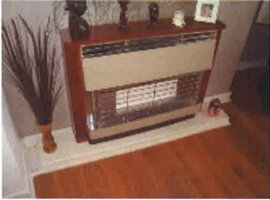
GAS FIRE WITH BACK BOILER
