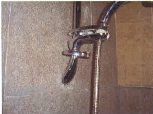
BROKEN SHOWERHEAD BRACKET WASHING MACHINE
