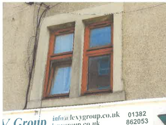
4. Living room windows external view.
