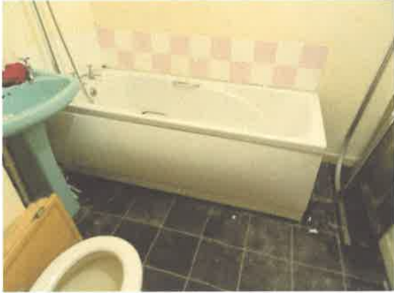
5. Replacement bath panel
