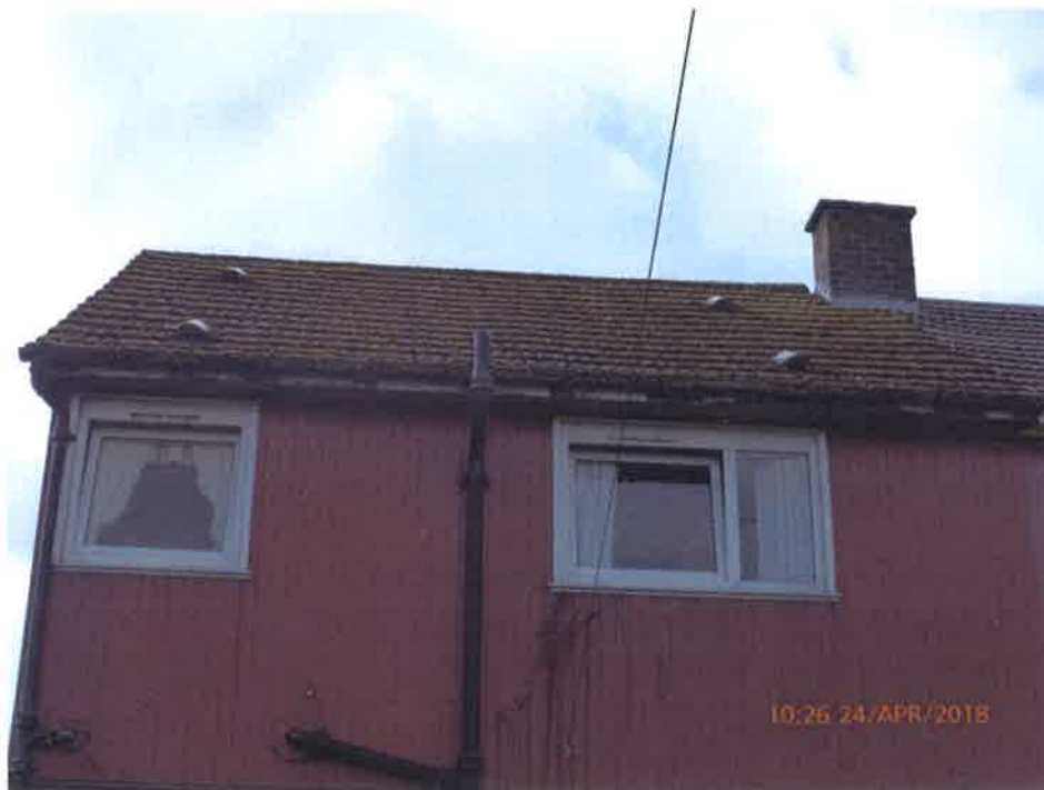
Rear roof detail
