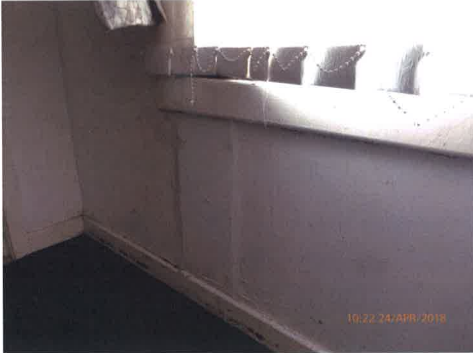
Repaired wall in the living-room
