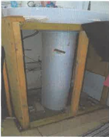
Photo 8 – Unfinished boxing of sink unit
