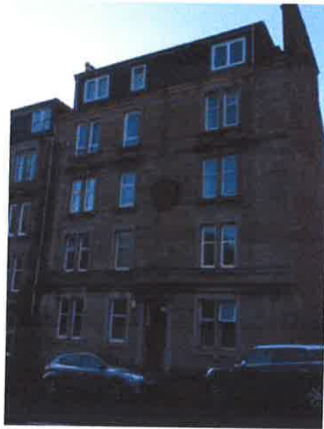
Ground floor flat – front elevation – 28 September 2017
