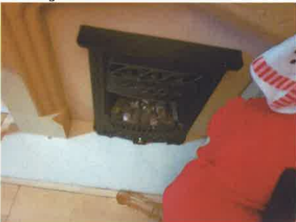
29 Gas fire – unable to be tested.
