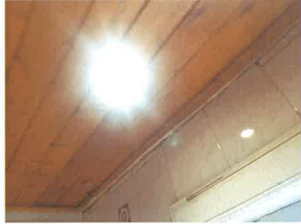
8 Bathroom spotlights operational.
