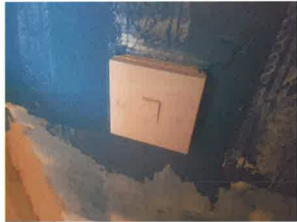
10 Light switch to Liam's Bedroom replaced and operational.
