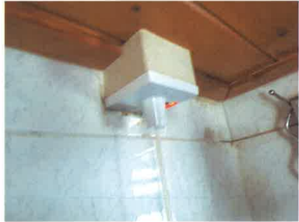
4 Electrical pull cord replaced.
