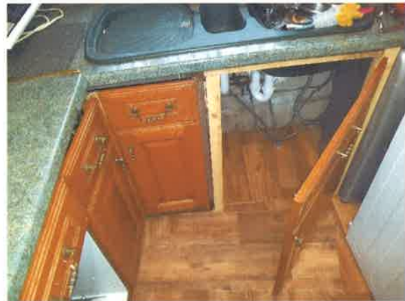
24 New kitchen flooring.
