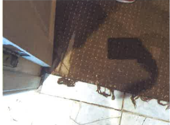
32 Damage to carpet at bathroom threshold.
