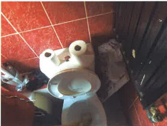
5 Toilet flush replaced.
