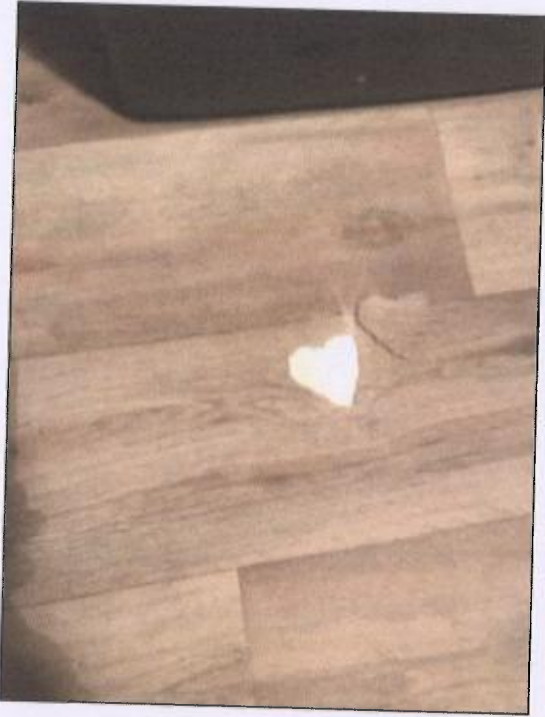
Vinyl flooring damaged in sections
