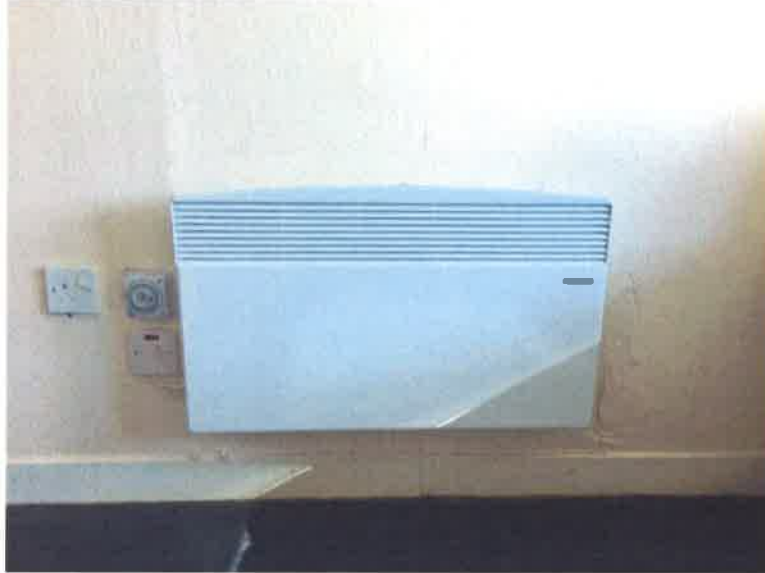
Living room – replacement heater – 6 April 2017
