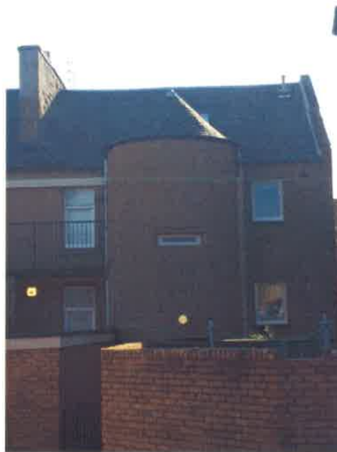
Mid Road elevation – 6 April 2017
