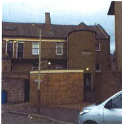
Mid Road elevation – 13 September 2016
