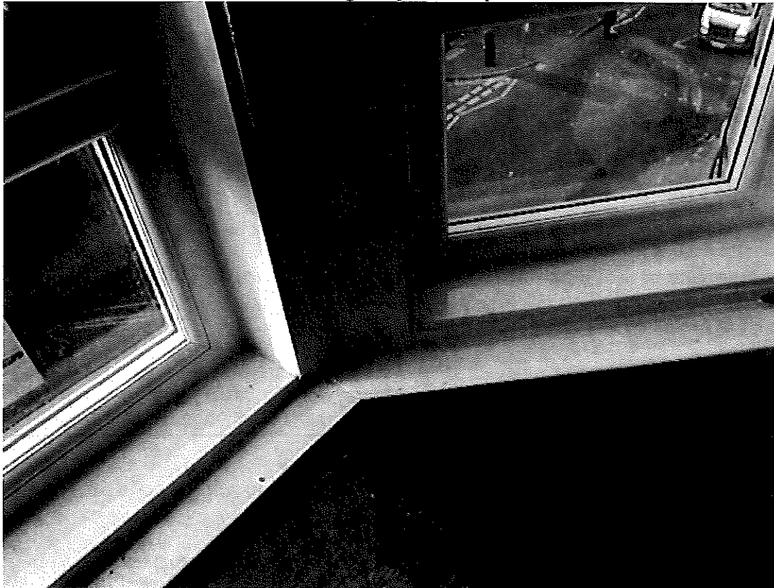
Partial view of area of window lining subject of repairs
