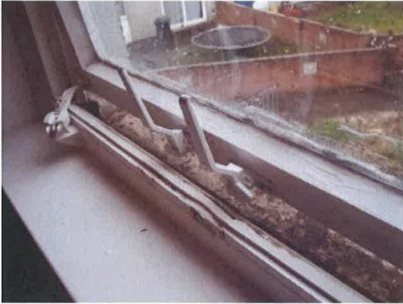
Open window showing draughtproof strips.
