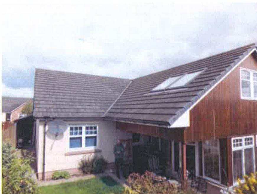
Rear of house showing conversion
