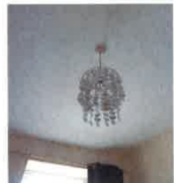
4. Repaired bedroom pendant light fitting
