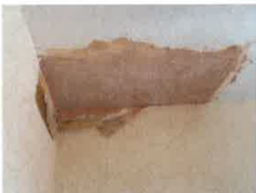
2. Plaster repair to bedroom ceiling
