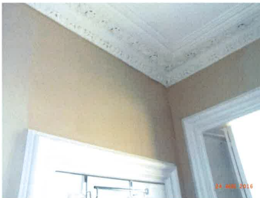
Bedroom 2 (Room south west) – Upper wall/cornice/ceiling
