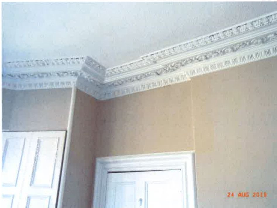
Bedroom 1 (Room north west) – Upper wall/cornice/ceiling
