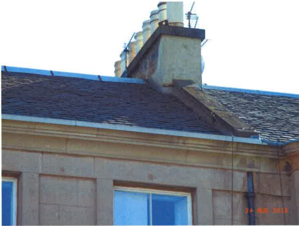
Roof/Chimney detail – Front elevation south
