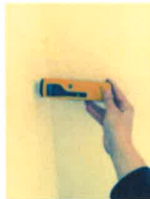
Damp meter reading – front bedroom (right hand wall)
