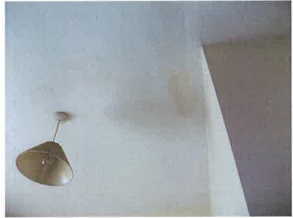
08 - Rear bedroom - dampness at ceiling (On internal wall and possibly from the flat above)
