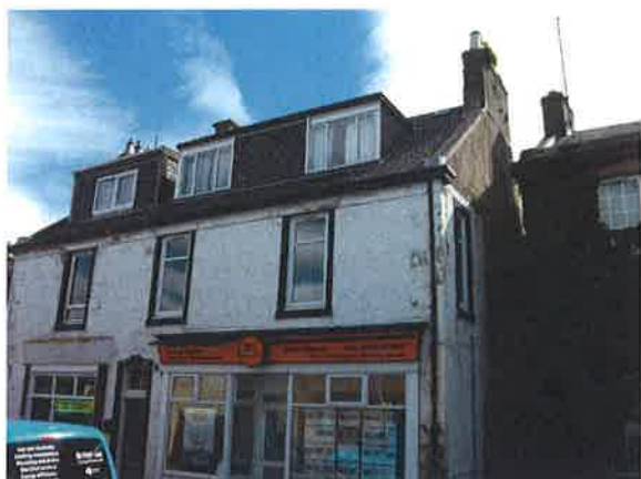
01 - Front Elevation (First floor flat, above 24-7 property shop)
