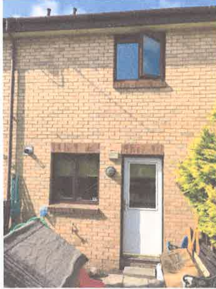
Rear elevation of house
