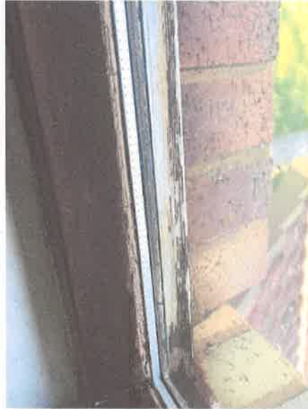
Close up of window frame
