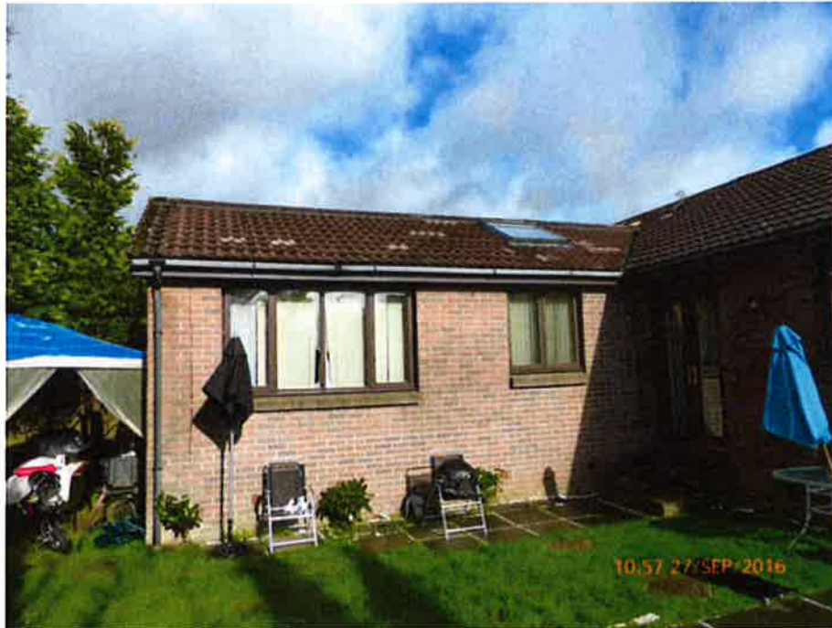
Rear, showing replaced tiles
