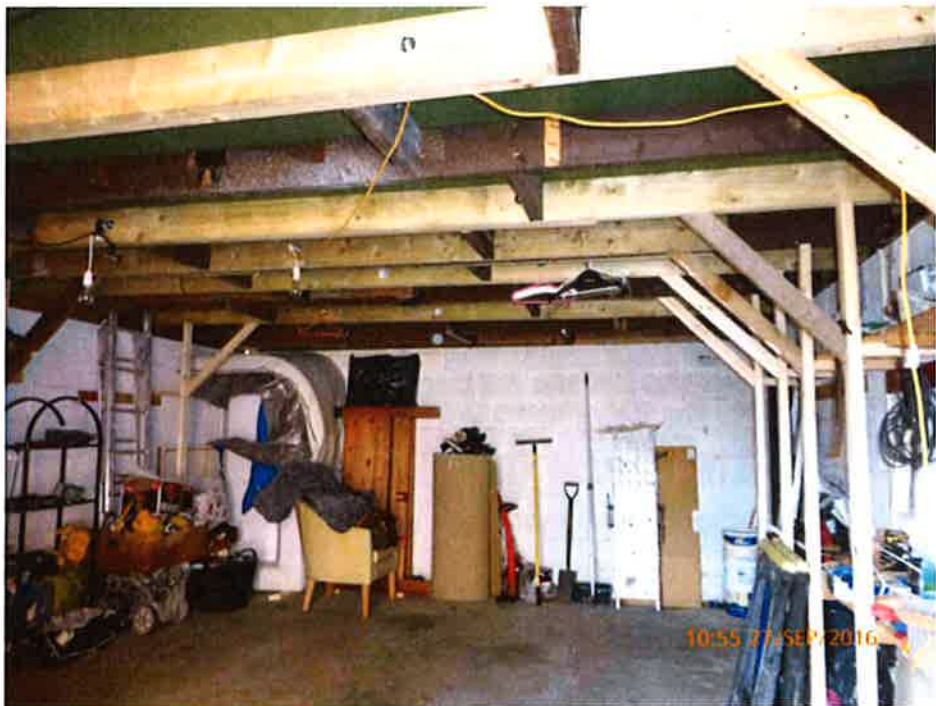
Interior of garage showing new roof and support
