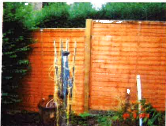
New fence in rear garden
