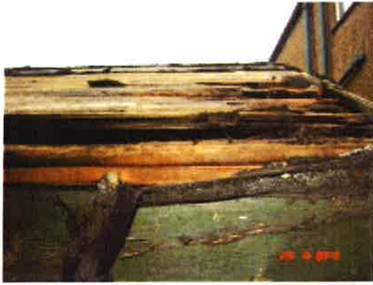
Roof of garden shed.
