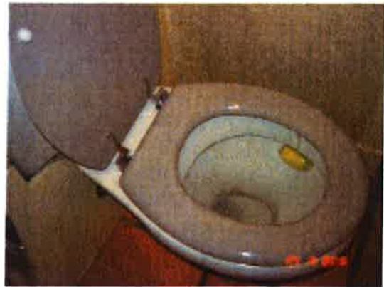
New toilet seat
