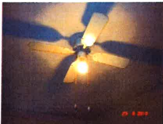
Ceiling fan/light in Living Room
